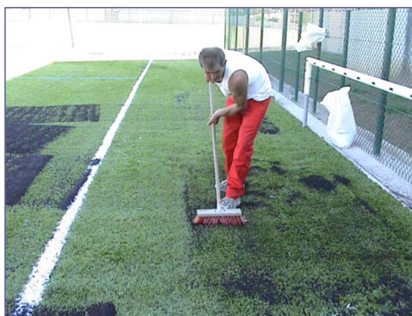
Figure 3: Installation of a roll of artificial fibre turf to cover the lysimetric system.
